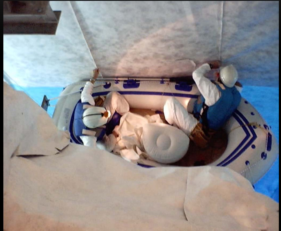
Alec Habig (UMD) and Jim Stone (BU), fixing Tyvek in barrel of OD
