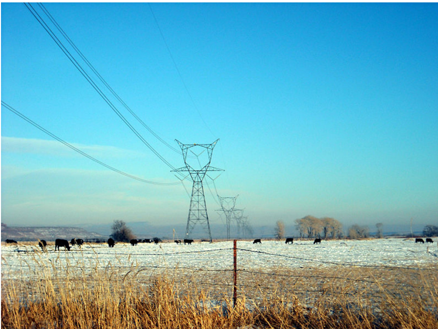
High Voltage Transmission line pic from Wikipedia
